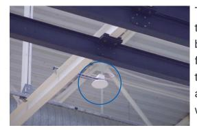
The antennas fixed on the top will cover a maximum of the ground surface, in order to detect all the surrounding beacons and thus calculate the angle of arrival of the signal formed between them and the beacons. The beacons will then transmit the positioning information to the business application through the **Quuppa Positioning Engine tool** which will transform the raw data into GPS data.
